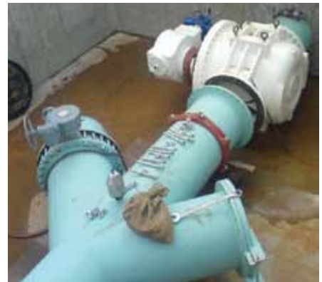
48" (1200mm) Model R-88 couplings used in a water treatment plant, Quarry, Utah, USA
